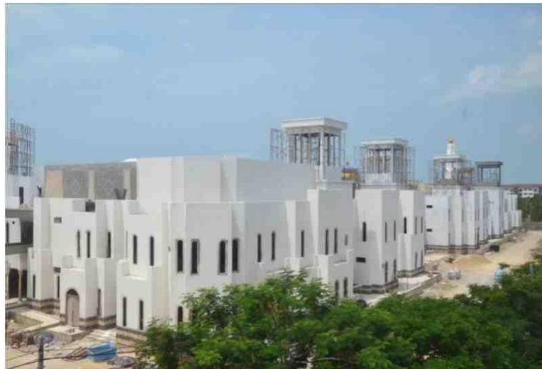
Figure 2. The Failed Arab City Project 16
